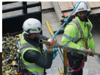
Over 200 site operatives
