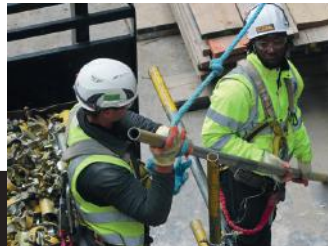
Over 200 site operatives
